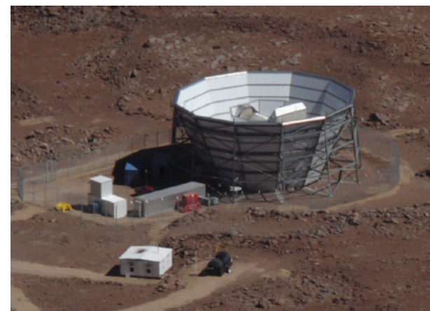
Fig. 1. The Atacama Cosmology Telescope, one of the many specialized instruments now being used to map the CMB. It is almost hidden behind the 12-sided shield placed to prevent radiation from the ground leaking into the telescope. (Image credit: ACT Team)
