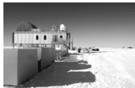
Taking out the trash. The line of cardboard boxes on the left are for sorting trash. All garbage has to be shipped back to Washington state in order to protect the delicate Antarctic environment. The boxy building at the rear houses the AST/RO submillimeter telescope. It is up on stilts so that drifting snow can slide underneath rather than piling up and burying the building. Photo © 1994 Maohai Huang. Used by permission of Maohai Huang.
