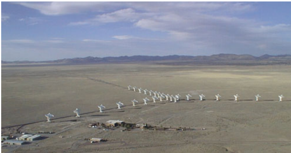
Aerial view of the Very Large Array, looking north-northeast. This set of large radio telescopes is used for a variety of astronomical observations including SETI searches. Here the antennas are in their closest configuration (D configuration). Photo by Dave Finley: Courtesy NRAO/AUI
